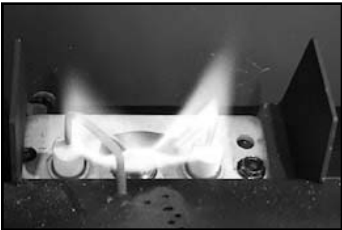
Figure 4.2 IPI Pilot Flame Patterns
