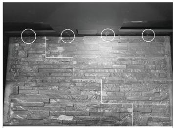
Figure 8.4, Back Refractory Panel Installed
