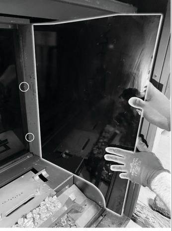
Figure 8.6, Side Black Glass Panels Installed
