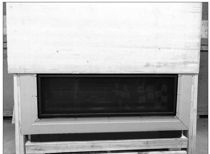
Figure 4.8, Installed Panels and Non-Combustible Material
